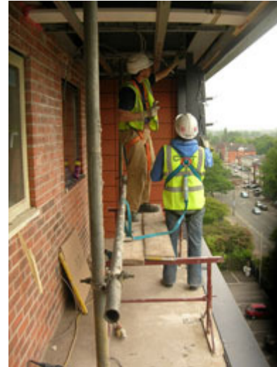
The two workers on the Options Properties Ltd site
