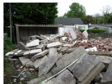
The IBT Contracting Ltd demolition site
