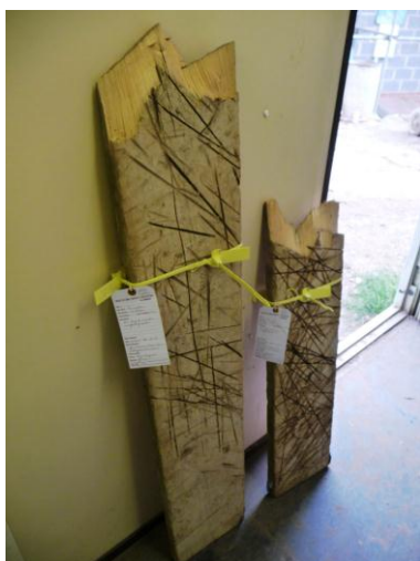
The broken scaffolding plank
